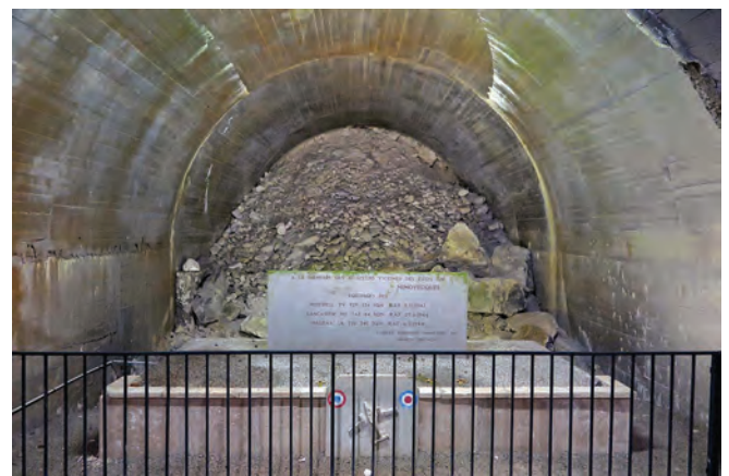
Memorial to RAF crews lost whilst bombing the site, evidence of their work behind. Photo Bob Clary
